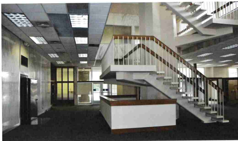
Lobby looking east
